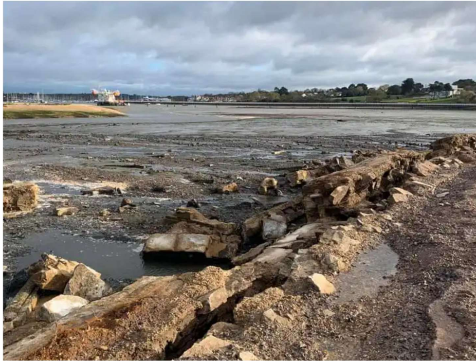
Figure 8: Hook Lake sea wall collapse (Source: Coastal Partners)
