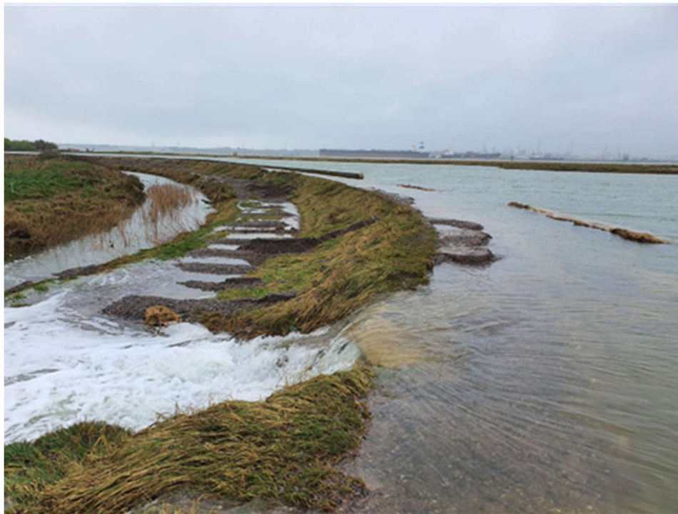
Figure 9: Hook Lake sea wall collapse (Source: Hampshire Highways)
